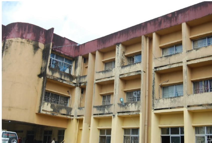
Fig. (2). The front of the teaching hospital (right wing) pre-renovation.
